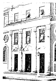
Entrance to "New" UI Chemistry Building profiled in AXE Hexagon (ca. 1930)
